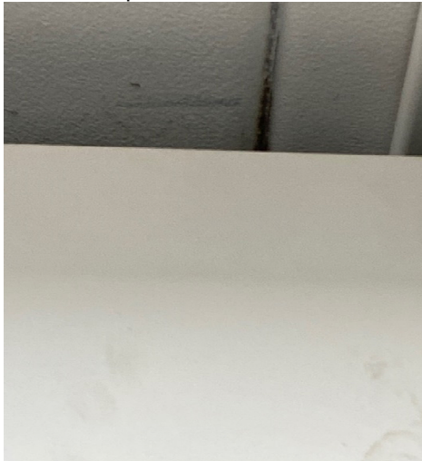
Dirt on HVAC Diffuser and Ceiling Tile – Upper Level
