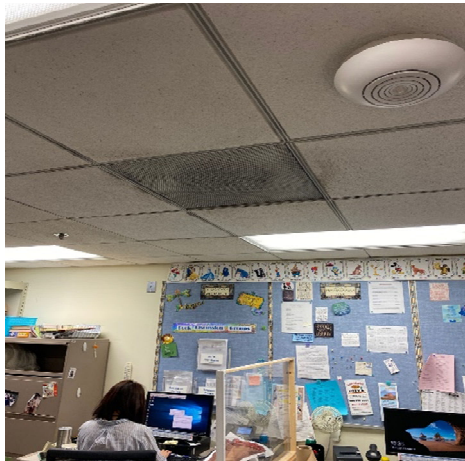
Dirt on HVAC Diffuser and Ceiling Tile – Upper Level
